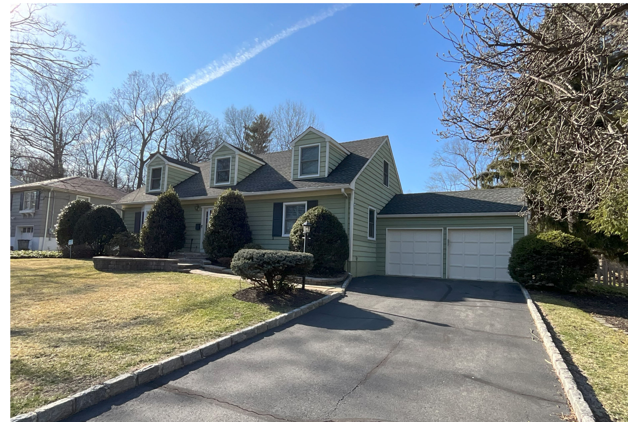
View of right side of house - Photo by Francesco Campo - 3.13.25
