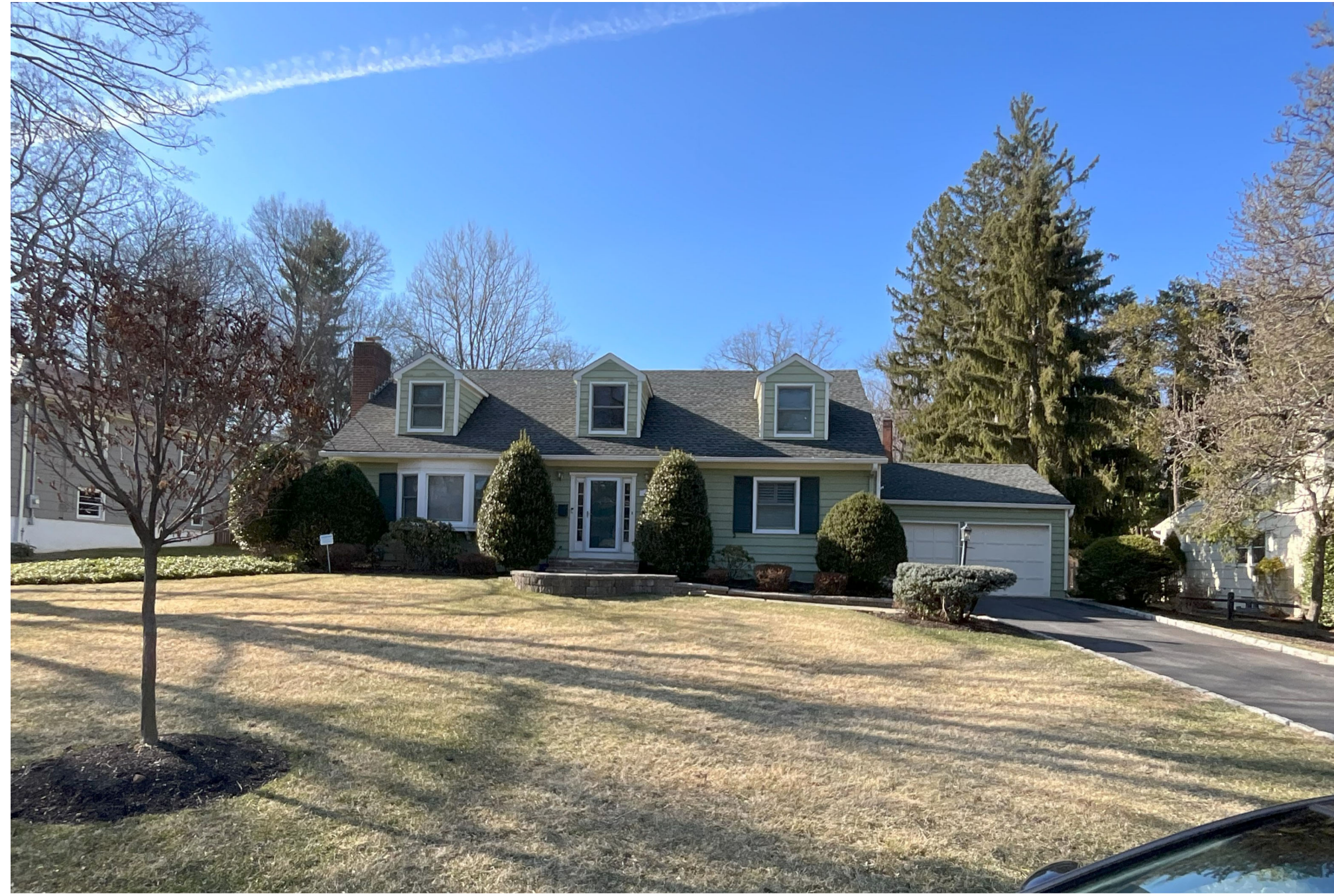
View of front of house - Photo by Francesco Campo - 3.13.25
