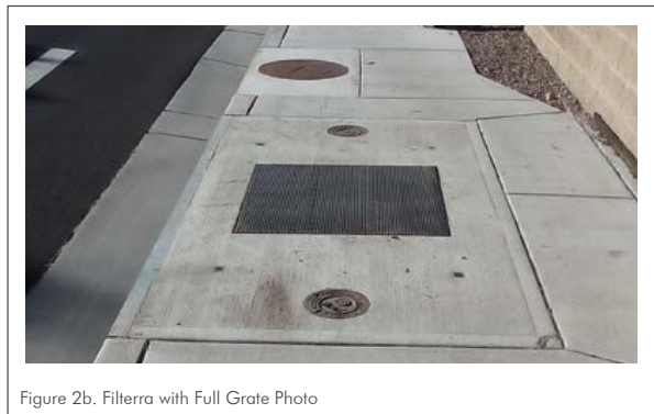
Figure 2b. Filterra with Full Grate Photo
