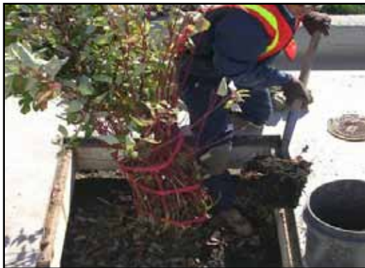
3. Removal of debris, trash and mulch
