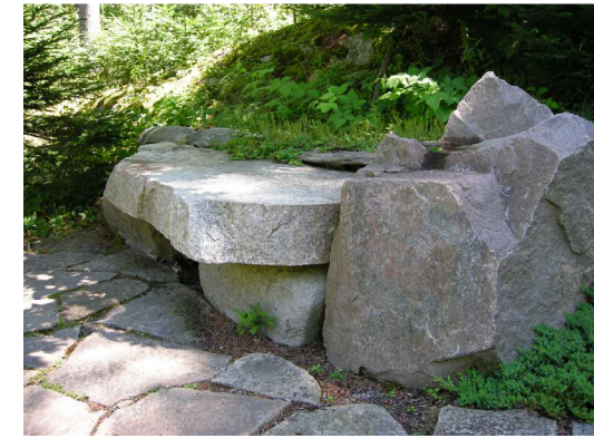
REFERENCE IMAGE NOTE: PROVIDE REGIONALLY-SOURCED TRAP ROCK (BASALT) MATERIAL; FIELD DRESSED AS REQUIRED TO PROVIDE FLAT, LEVEL SEATING SURFACE.
